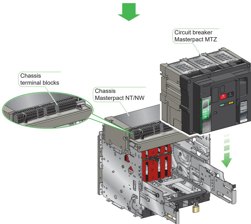
Specific attention of the MasterPact NT/NW chassis condition is required prior to proceed with breaker replacement.
