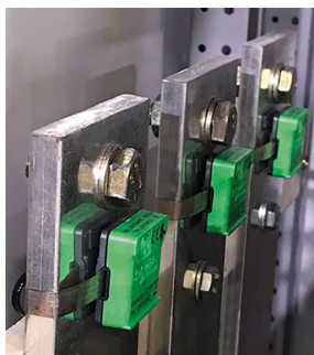
Connection Temperature Monitoring
