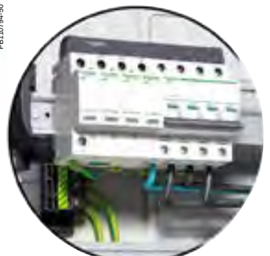
Surge arrester iPRD 4P + iC60N 4P
