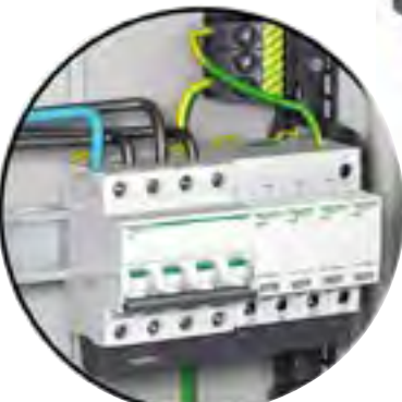
Surge arrester iPRD 4P + iC60N 4P
