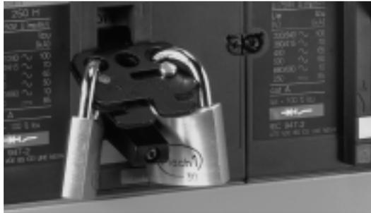
**fig. 23:** Padlocking device on a Merlin Gerin Compact circuit breaker.
